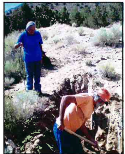
Reano Castell and Peter Foust begin digging the trench for the new water pipeline.
