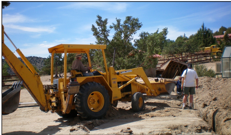
The Reverend Ted Staver operating a bulldozer to dig a trench for the new water pipeline at the Red Rock Consecrated Sanctuary with Steve Larson assisting.
