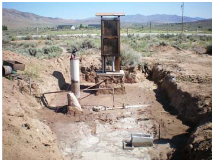
The existing well head. PHOTO: Ted Staver
