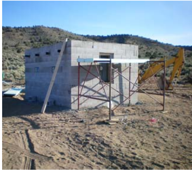
Main structure of Argonaut pump house under construction. PHOTO: Ted Staver
