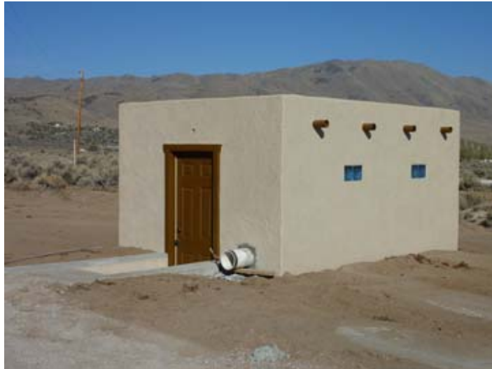
Completed pump house on Argonaut Way. PHOTO: Ted Staver
