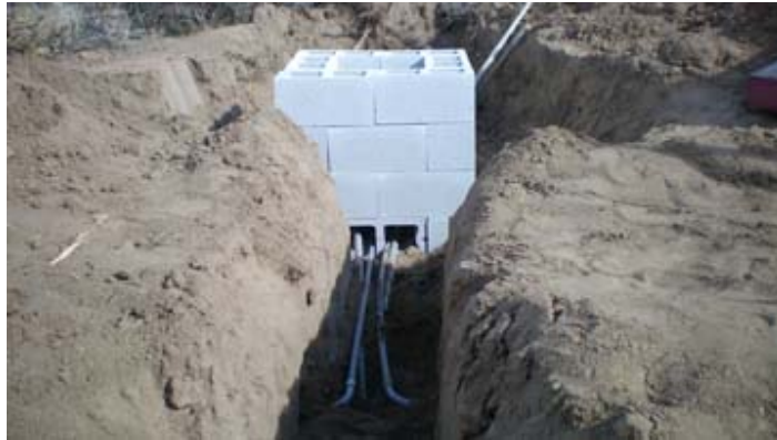
Last pull box. PHOTO: Ted Staver
