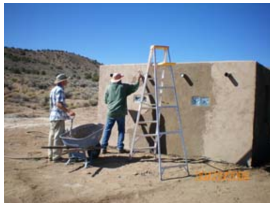
Argonaut pump house being finished with stucco. PHOTO: Ted Staver
