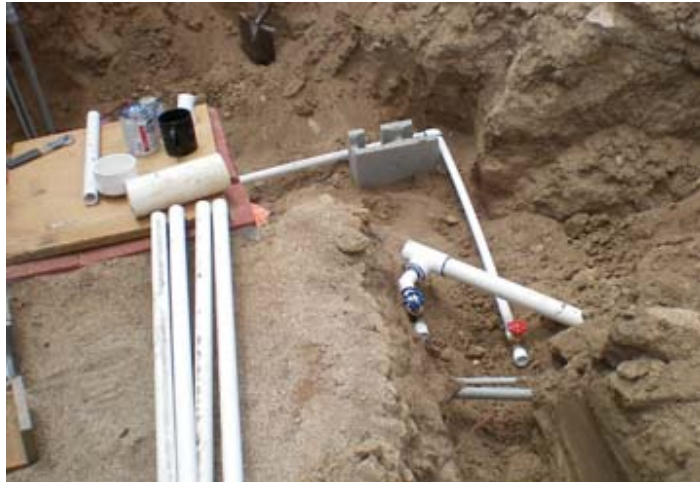
Pipe laid near the lift pump station. PHOTO: Ted Staver
