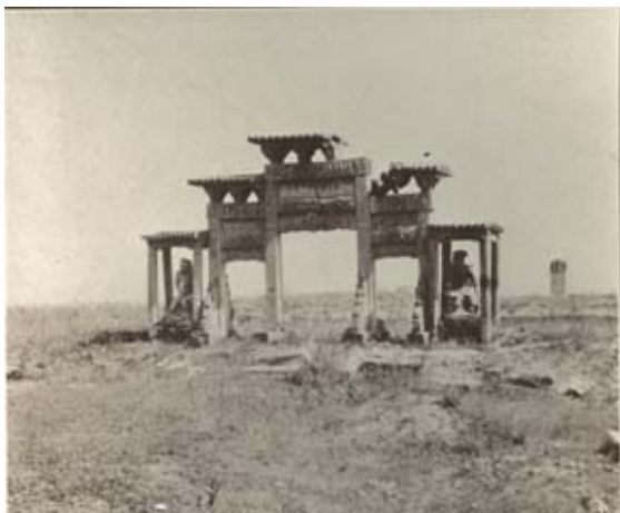
Arched stone gateway in ruins
