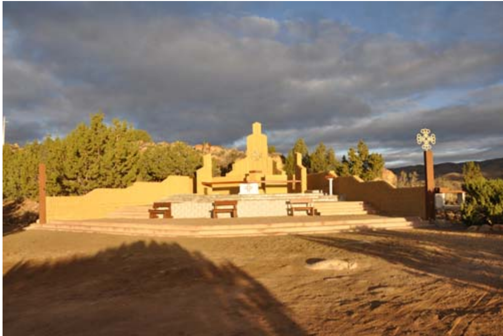
Church of New Epiphany after 2013 renovations. PHOTO: Stephan Fuelling
