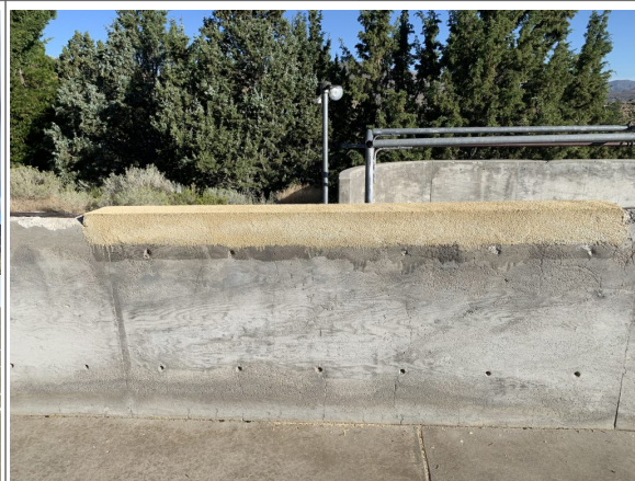
Wall during phase 2 of repairs
