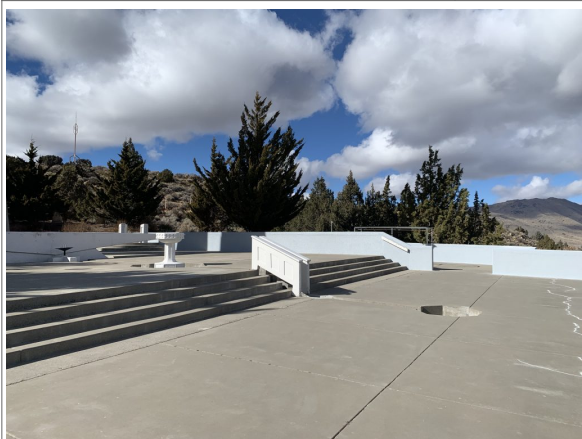
Vestry Walls repairs complete
