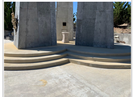
Triune Cross Base repairs nearly completed
