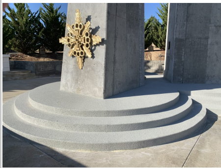
Triune Cross Base repairs complete
