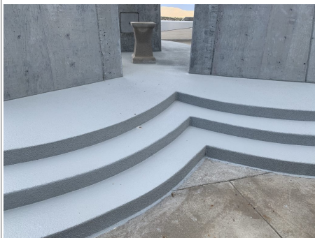
Triune Cross Base repairs complete
