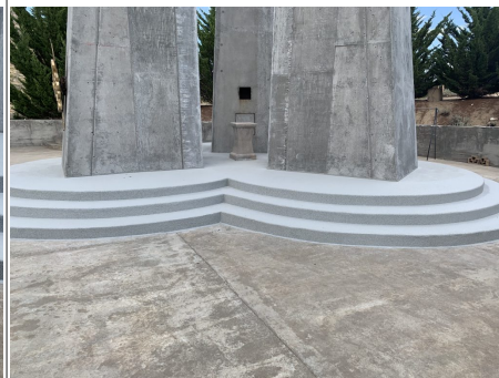
Triune Cross Base repairs complete
