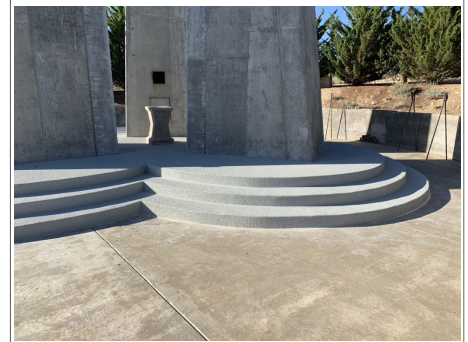
Triune Cross Base repairs complete
