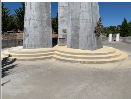
Triune Cross Base repairs nearly completed
