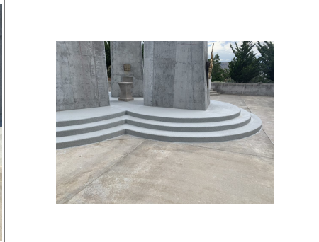
Triune Cross Base repairs complete
