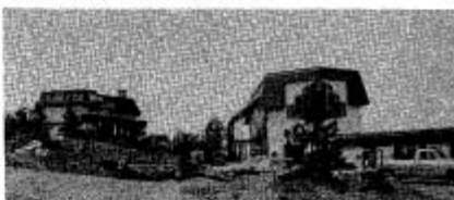
The existing Rectory-Abbey of Bishopstead with "East Wing" addition near completion
