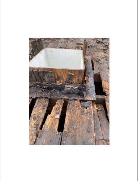
At least four layers of old roofing had to be removed to get to the original wooden structure, which dates to 1927 when the older bathhouse was rebuilt after a fire destroyed it. In many
