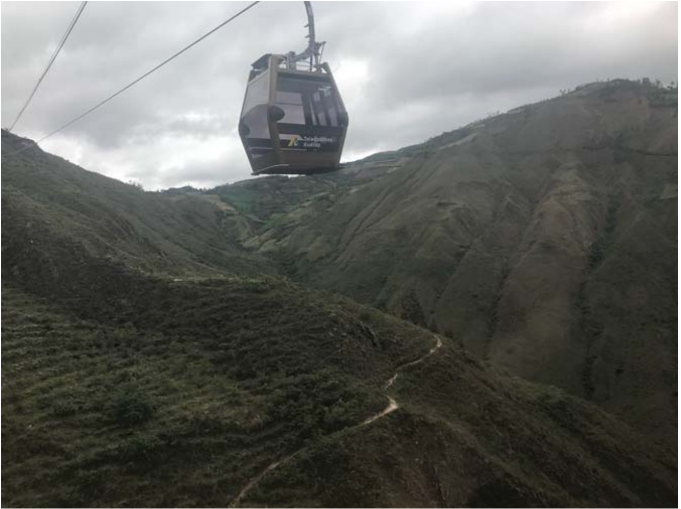
New cable car tramway with old mule trail below
