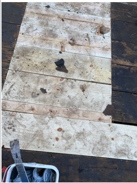
At least four layers of old roofing had to be removed to get to the original wooden structure, which dates to 1927 when the older bathhouse was rebuilt after a fire destroyed it. In many
