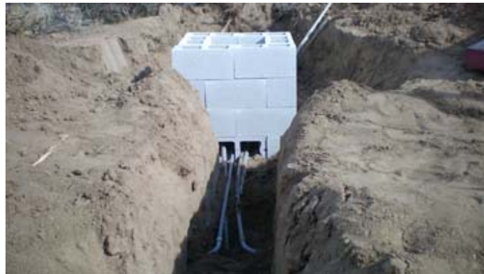
Last pull box. PHOTO: Ted Staver
