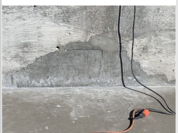
<Crumbling Lower Wall After repair>
