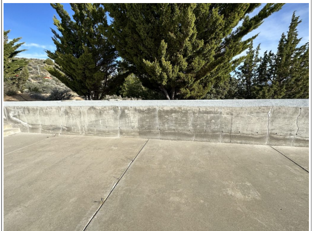
<Crumbling upper wall After repair >
