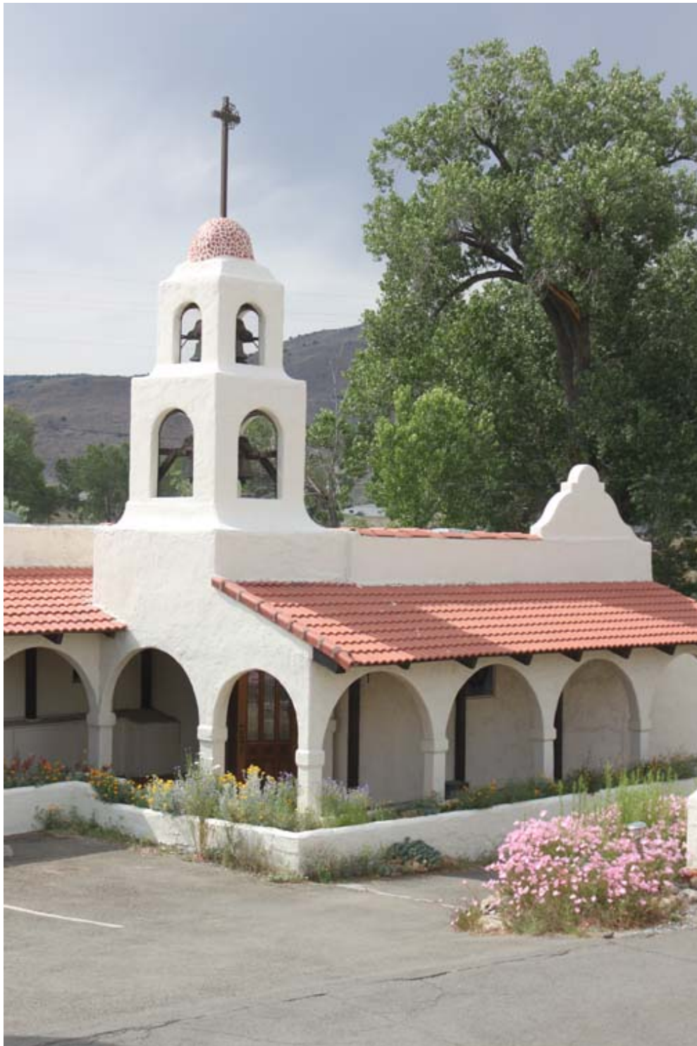
Steamboat Chapel of the Roses exterior after 2015 renovation PHOTO: Muriel Cervantes
