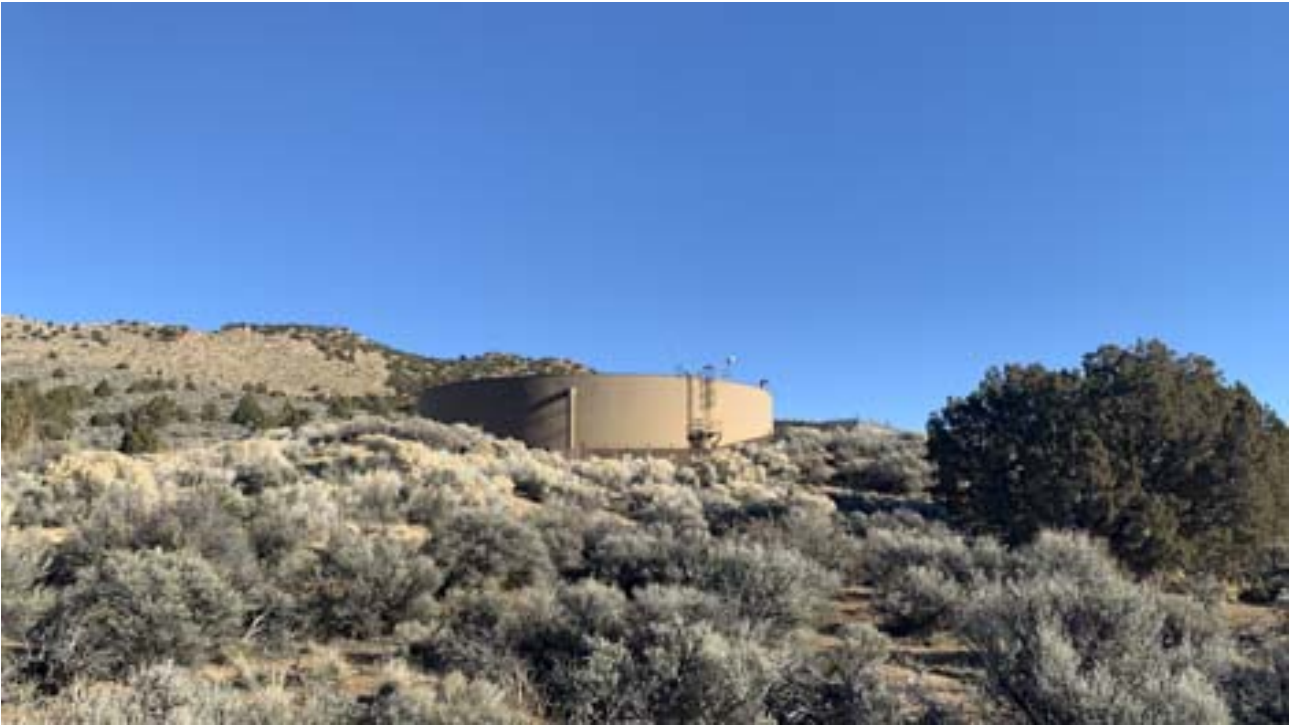
TMWA's 2 million gallon water storage tank
