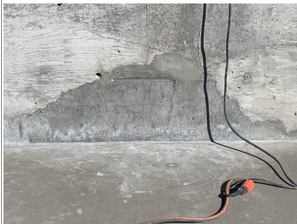
<Crumbling Lower Wall After repair>
