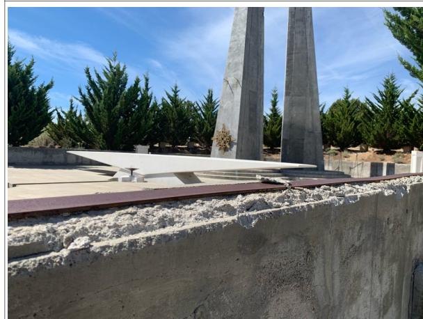
<Crumbling upper wall After repair >
