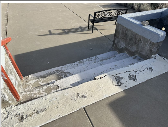
<Crumbling steps at the Bell Choir After complete repair>
