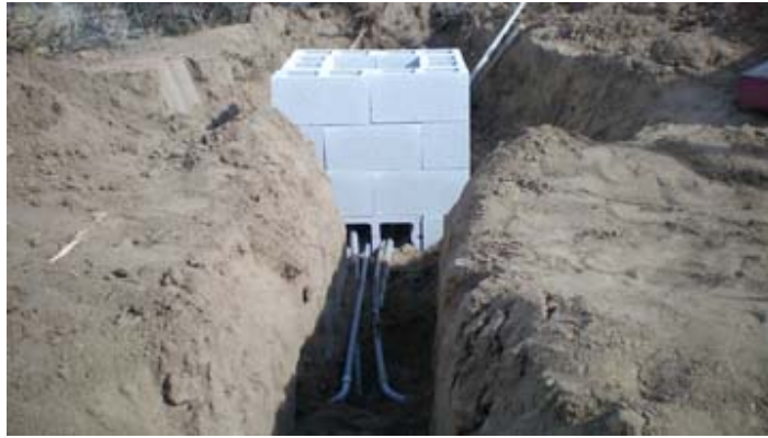
Last pull box. PHOTO: Ted Staver
