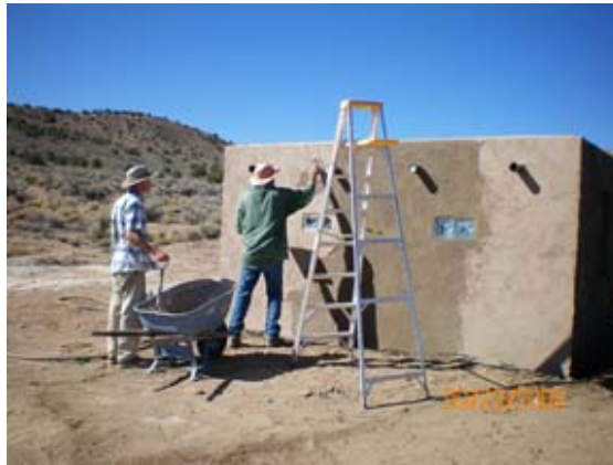
Argonaut pump house being finished with stucco.
