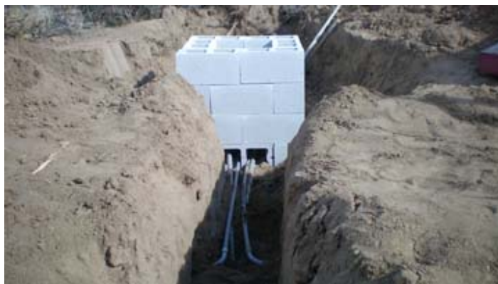
Last pull box. PHOTO: Ted Staver
