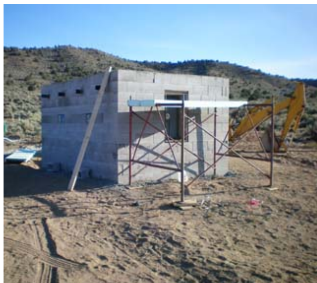
Main structure of Argonaut pump house under construction.
