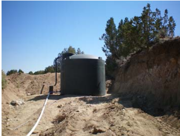
Water tank set up between pond and lift pump station. PHOTO: Ted Staver
