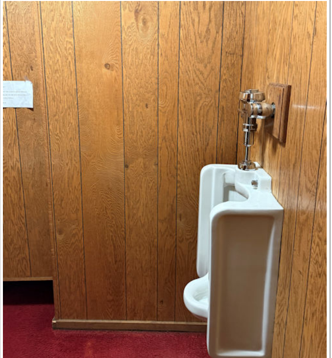
Chancellery Men's Washroom
