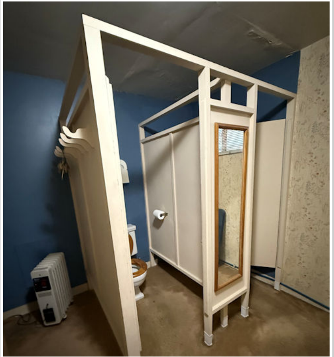
Chancellery Washroom Ladies
