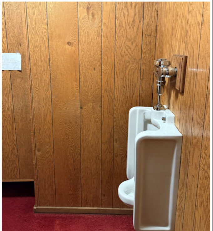
Chancellery Men's Washroom
