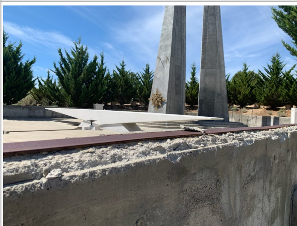
<Crumbling upper wall After repair >
