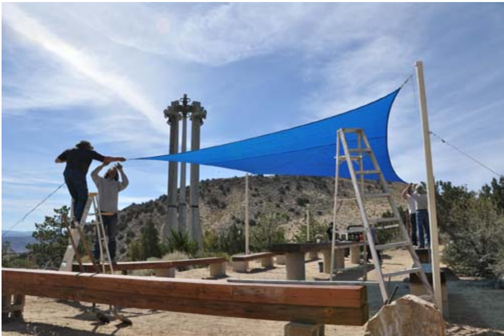
Michael McIntyre, Ted Staver, Robert Roy and Sean Savoy help assemble new Refectory covering.
