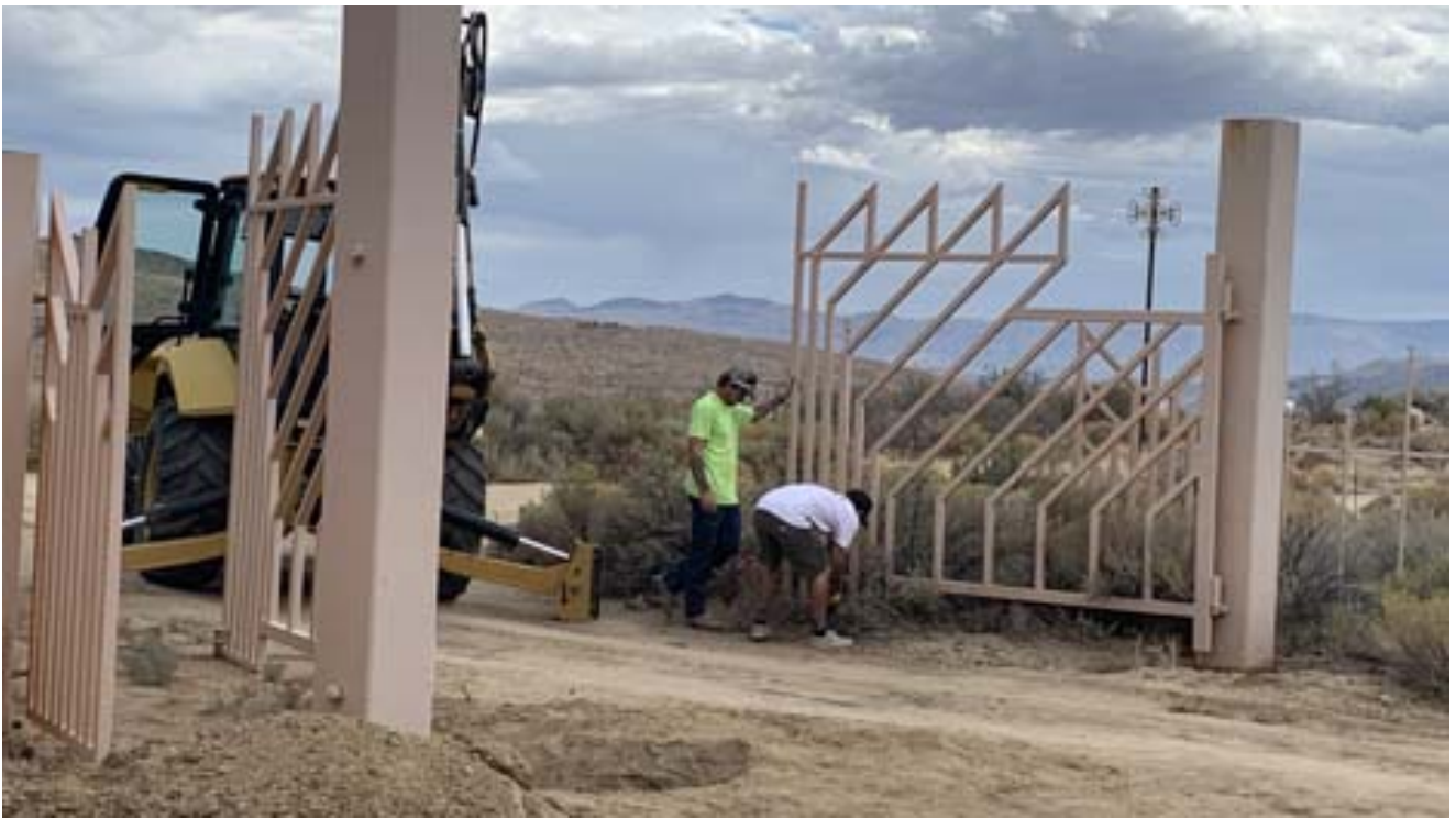
Work begins with the removal of the Zion gate.
