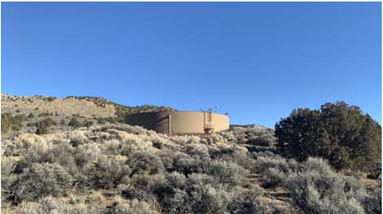
TMWA's 2 million gallon water storage tank
