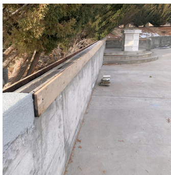
Ongoing Repairs at the Cathedral
