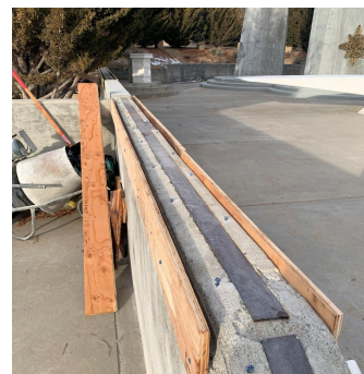
Ongoing Repairs at the Cathedral
